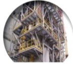
OTHER PROCESSING EQUIPMENT
